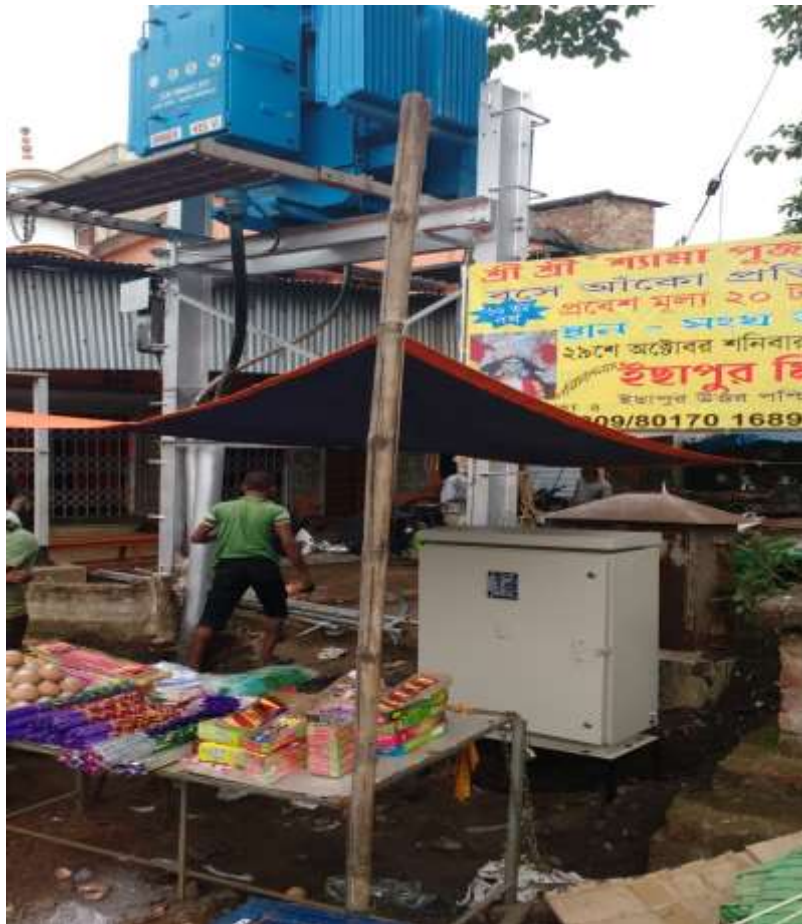
APFC Unit installed at Sealdanga (C) P/T
