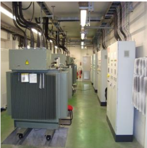
European Synchrotron Radiation Facilities 14 x 800 kVA @ 20kV
