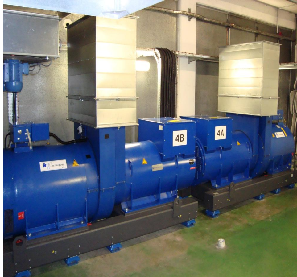
European Synchrotron Radiation Facilities 14 x 800 kVA @ 20kV
