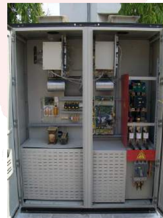
STATCOM – Load Balancer / 1Ph Statcom 440V, 100kVA
