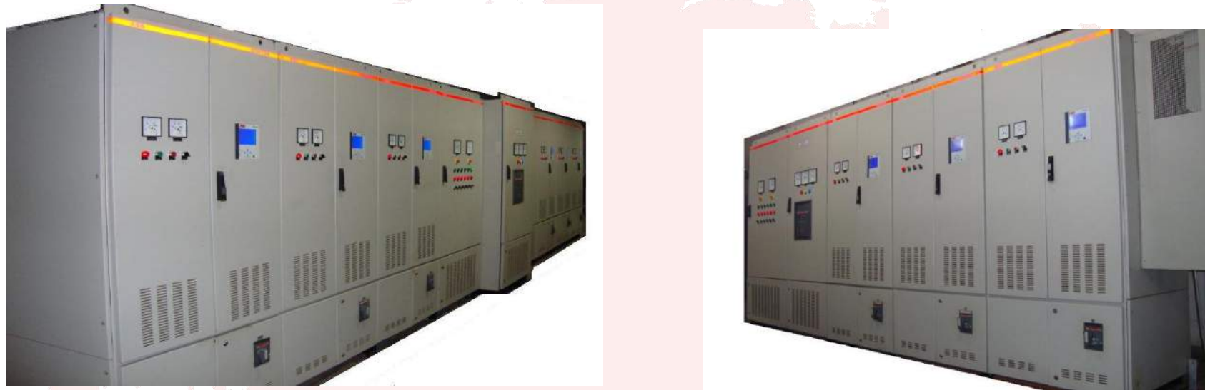
Figure 21 : PQC Installation in M/s FIAT India Automobiles.
